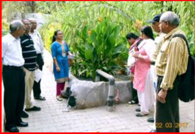
Visit to Sewage Treatment Plant at the Hostel of College of Engineering, Pune
